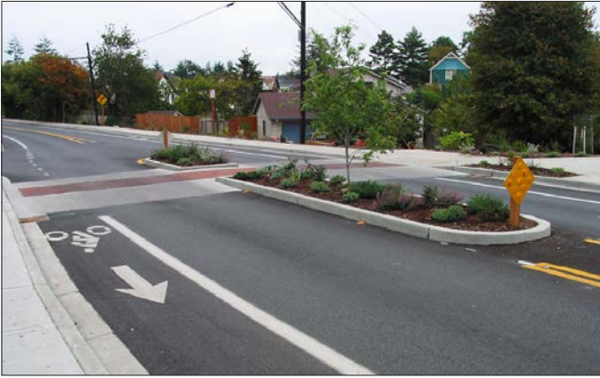
Median refuge islands are protected areas where pedestrians, who may be less able to cross the street in one stage, may safely pause or wait while crossing a street.
