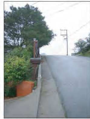
Steep grade at 20 River Oaks Road. Sidewalk construction may require retaining wall.
