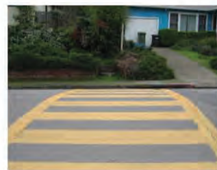
Looking southwest across 5th
