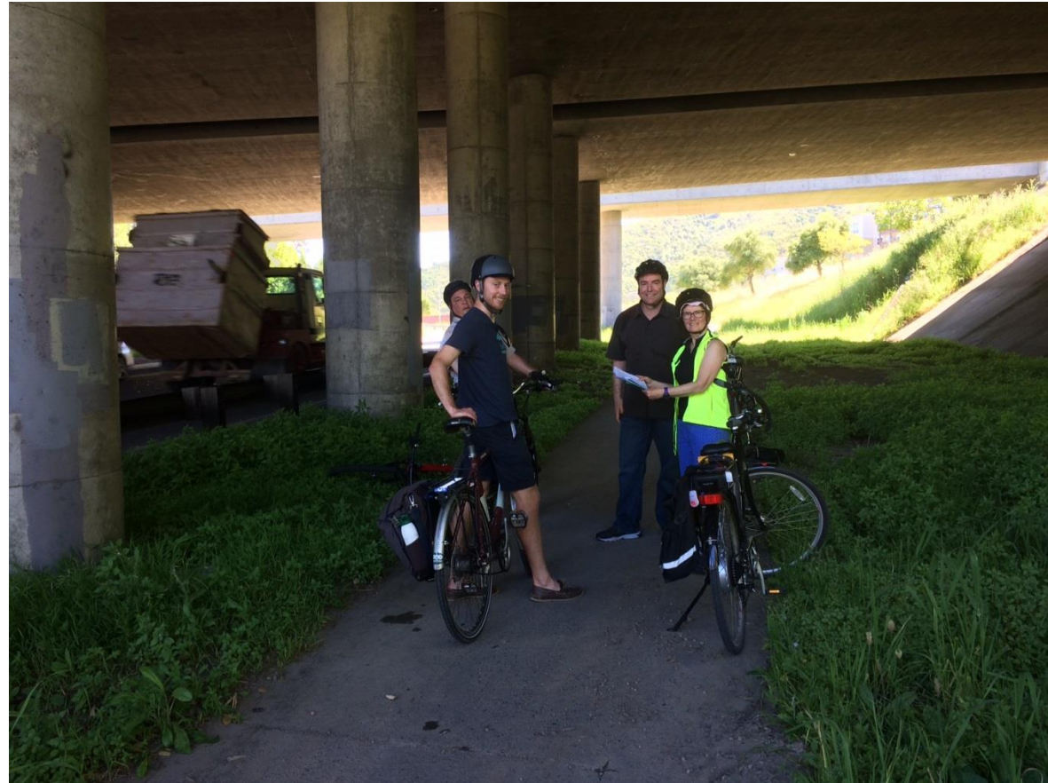
Hwy 101 Undercrossing at N. San Pedro Rd. Path exists, needs minimal work to upgrade to pleasant Class I facility. Challenges exist at Caltrans on/off ramps outside photo.
