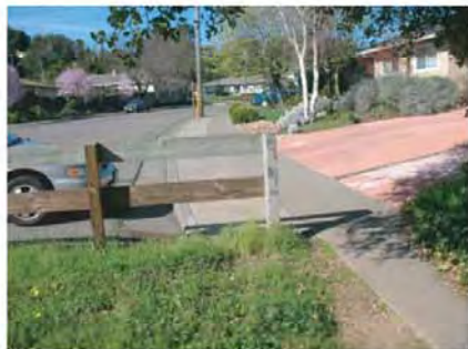
Existing sidewalk and fence
