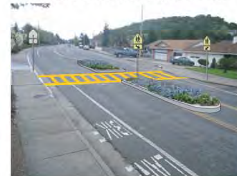
AFTER: Pedestrian refuge installed
