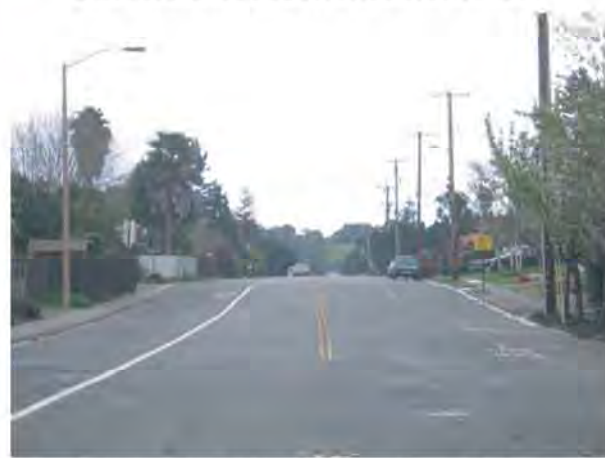
Typical cross section of Olive Avenue, showing 13 ft shoulder
