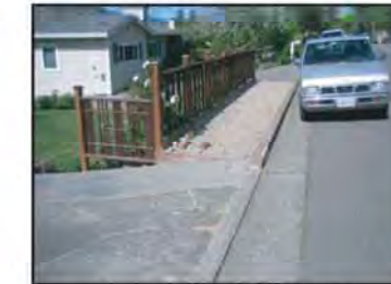
Steeply sloped driveway
