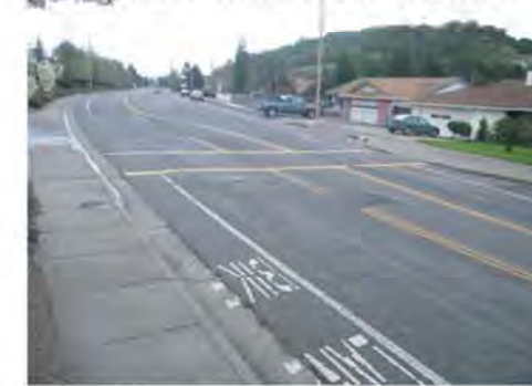
BEFORE: Crosswalk in front of school
