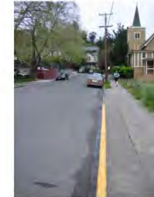
South curb of Old Mill
