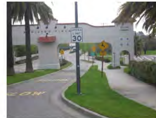
Facing east on Main Gate Road 30 mph sign is placed before school sign clutter distracts
