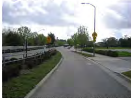
Approaching crosswalk from west on Main Gate Road
