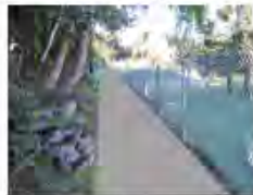
Widened paved path
