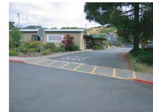
Crosswalk in front of school parking lot entrance
