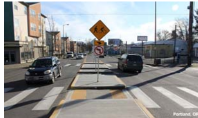
Median refuge island
