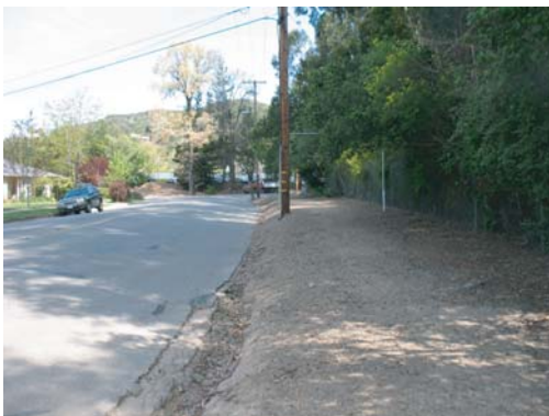
Looking north on Belle Avenue showing elevated berm
