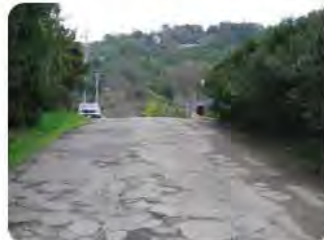
Looking southeast up Berkeley toward Brookside Dr.
