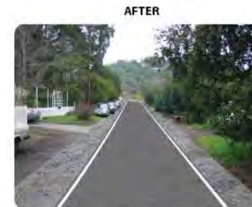
16 foot pavement with gravel parking area on sides
