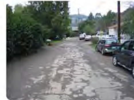
Looking northwest toward the school path entrance
