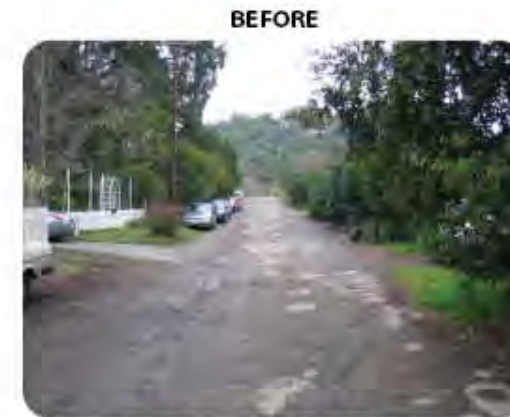
Looking southeast down Berkeley Ave. toward Broadmoor
