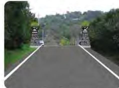
Gateway monuments at entrance, new paving
