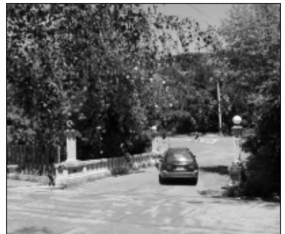
Manor Bridge will get a companion pedestrian bridge
